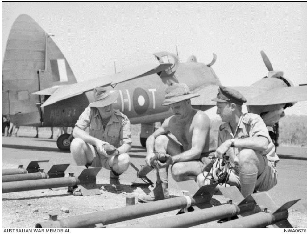
Figure 2 – RAAF personnel examine 3 inch 60lb HE or SAP warheads about to be fitted to rockets and loaded on the Beaufighter bomber aircraft - Coomalie Creek, NT, 1944 (AWM ID NWA0676)
