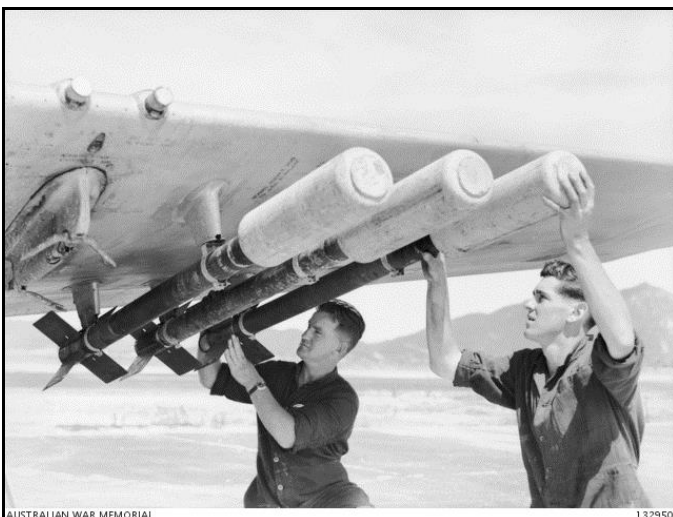
Figure 3 - RAAF personnel loading 60lb practice rocket bombs onto a P.51 Mustang fighter aircraft (AWM ID number 132950)
