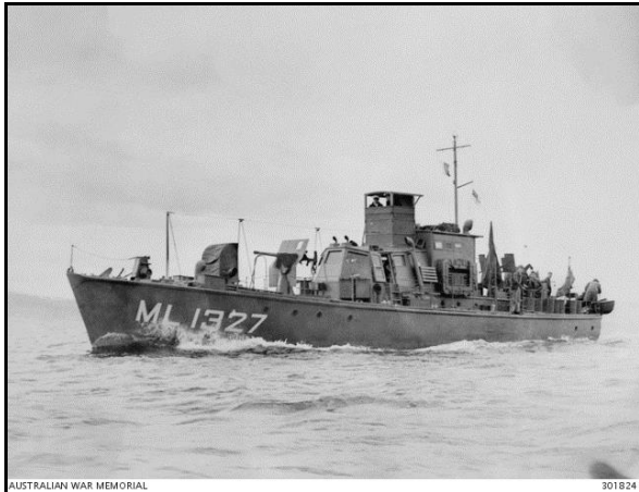
Figure 1 - HMA Harbour Defence Motor Launch (HDML) ML1327 with 3 pr gun mounted forward - Hobart, 1944 (AWM ID 301824)
